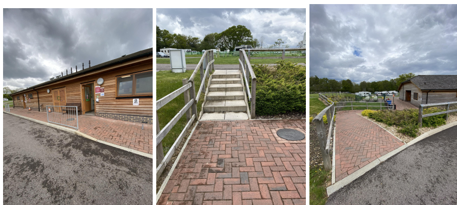
Dropped kerb, stairs and ramp to access the toilet block
