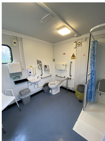
Accessible Toilet and Shower
