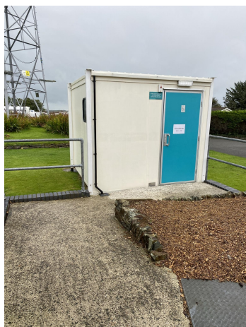
The Accessible Cubicle
