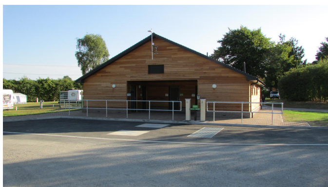
Upper Toilet Block
