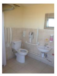
The **male and female toilets** have outward opening doors with clear opening widths of 750mm, with level entry. In both male and female toilets, each has an identified ambulant disabled accessible WC with drop-down and fixed grabrails. The privacy cubicles have lever taps to the washbasin, but no grabrails. There is no shower specifically adapted for ambulant disabled people, but one cubicle is wider at 850mm, and has level access between wet and dry areas.
