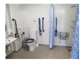
**Standard toilets** to the main Toilet Block are accessed via doors achieving a clear width of 885mm over a level threshold. Grab rails are provided to 1 urinal, a WC, basin and shower position. A shower seat is not provided. Taps and showers incorporate lever type controls. Showers have level access.
