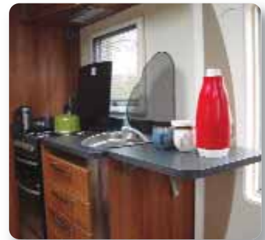
Hinged flap extends the amount of work surface available in the kitchen
