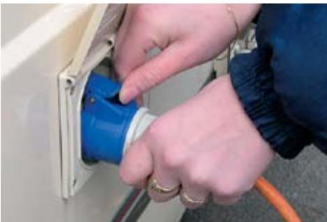
3. Locate your electricity supply bollard – ask the warden if you're not sure which one – and, ensuring the cable is routed out of harm's way, raise the cover on the individual outlet and insert the blue plug (male). On Club sites, turn the plug clockwise until it locks. On other sites you may simply need to push it home firmly.
