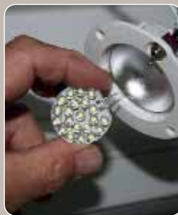
Some of the halogen lamps on ceilings and under shelves can be replaced with LED units
