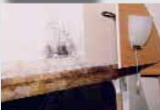
■ Have a close look at wall and ceiling panels for tell-tale signs of developing leaks. Harsh winters sometimes damage ageing external sealant.
