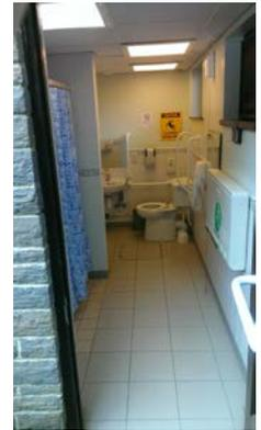
The combined **female WCs/showers** have four WC cubicles, none with grab rails. Open area washbasins have thumb turn taps. The area also has four privacy cubicles, with thumb turn taps to washbasins, and no grab rails. There are four shower cubicles, one of which has grab rails, suitable for ambulant disabled users. Each cubicle has solid doors, with easy to use sliding bolts, and the shower cubicles also have curtain separation between wet and dry areas, with a 50mm step.
