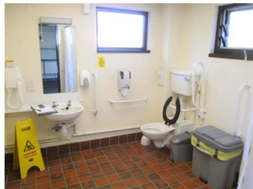
shower has no fold-down grab rail. The wash hand basin is located 750mm away from the WC pan, out of reach for some users. The cubicle is fitted with an alarm system.
