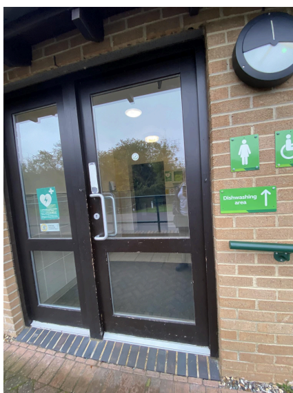
Door to the lobby
