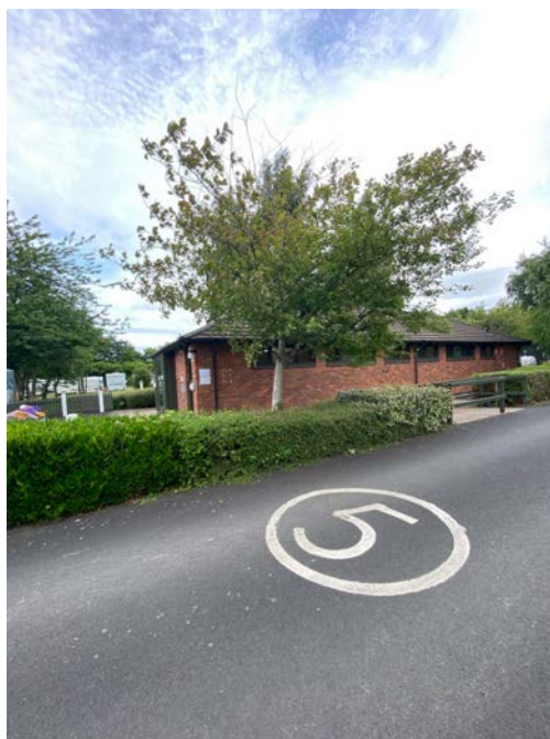
Toilet Block A
