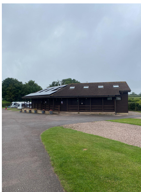
Black Rock Copse Toilet Block
