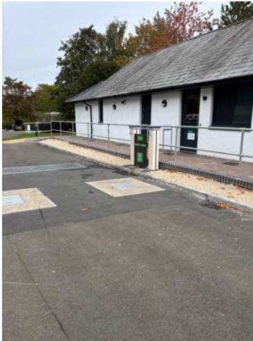
MHSP at Toilet Block A
