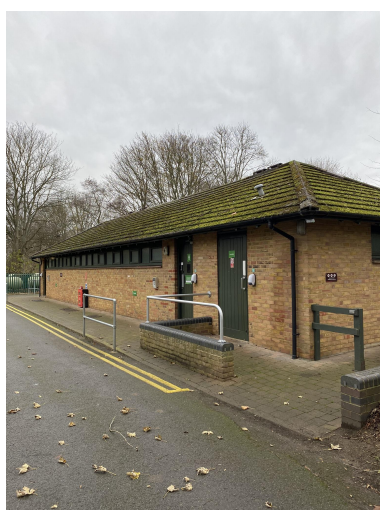
East Toilet Block
