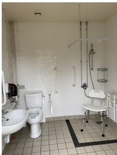
Accessible Toilet - East Block
