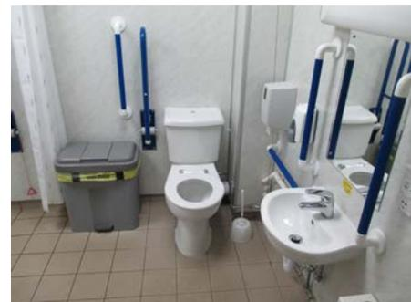
position. The cubicle is fitted with an alarm system. Whilst the width of the cubicle falls below best practice standards the cubicle does achieve a 1500mm wheelchair turning circle and there is sufficient transfer space adjacent to the shower and WC positions. The restricted manoeuvring space on entering the cubicle will make it difficult for a wheelchair user to open and close the door, which is not fitted with a horizontal grab rail.
