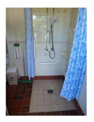
both male and female facilities, 1 toilet cubicle, 1 privacy cubicle and 1 shower cubicle have grab rails for support. The taps to the basins are lever type to assist people with limited manual dexterity.
