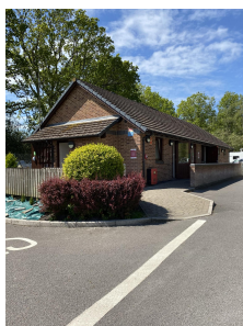
South Toilet Block
