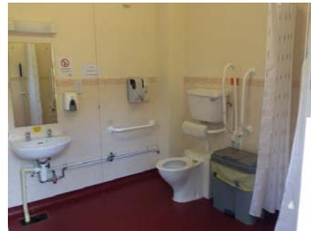
The **male and female toilets** have inward-opening doors with clear openings of 800mm. There is a 170mm step up into a lobby. The lobby has an outward-opening door with a 700mm clear opening. Both doors are stiff to open. In both male and female toilets, one shower cubicle, one privacy cubicle and one WC cubicle are fitted with grab rails. The taps to the washbasins are lever non-mixer. The accessible WC/shower is used instead.
