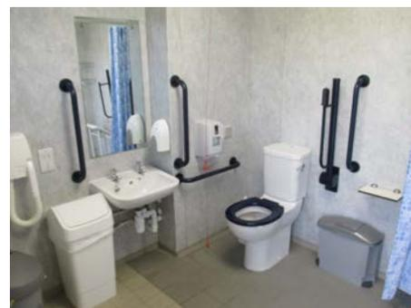
Toilet Block 2 **Male and female toilet** doors achieve an 820mm clear opening width over a level threshold. Ambulant disabled WC and shower cubicles are provided with contrasting grab rails. Shower cubicles are level access with a flush gully. WCs, basins and showers have ergonomic lever style controls.
