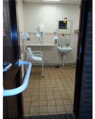
The **male and female toilets** have doors with clear opening widths of 740mm and stepped thresholds of 140mm and 130mm respectively; there are no grab handles at either door. The toilets both have lobbies and the doors are normally left open. In both male and female toilets, at least one shower cubicle, washbasin privacy cubicle and WC cubicle is fitted with grabrails to assist ambulant disabled people. The taps to the basins are lever type to assist people with limited manual dexterity.
