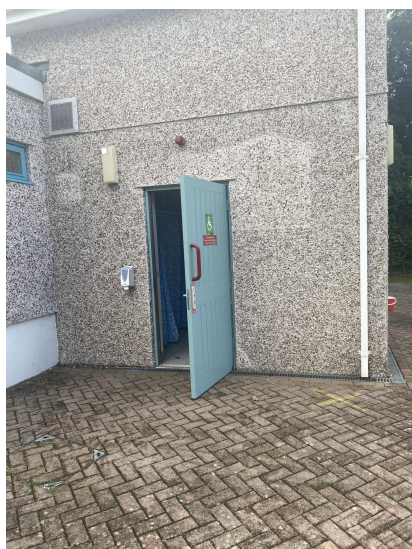
Entrance to Accessible WC and Shower Cubicle
