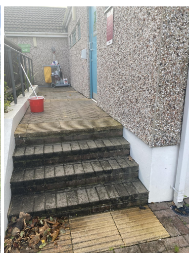
Steps around Toilet Block
