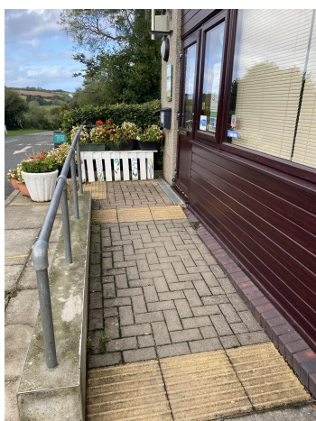
Ramp to reception
