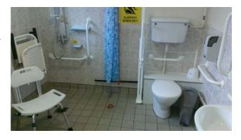
The **male and female toilets** have doors with clear opening widths of 780mm and flush thresholds, but they may be heavy to open for some people. In both male and female toilets, one shower cubicle, one washbasin privacy cubicle and one WC cubicle is fitted with grab rails to assist ambulant disabled people. The taps to the basins are lever type to assist people with limited manual dexterity.
