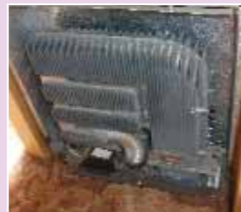
Fins on a heat exchanger inside a wall-mounted appliance efficiently release warmth into the living area
