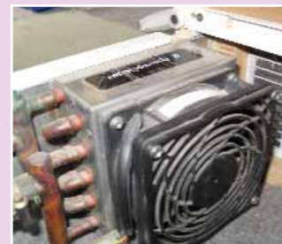
A fan blowing through a tiny radiator in this oil-fired heating system adopts a principle employed in car heaters
