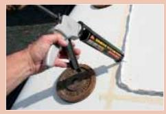
The roof is cleaned and the position of the panel marked with tape before caravan adhesive sealant is applied. This is placed around the perimeter and across the centre of the panel.
