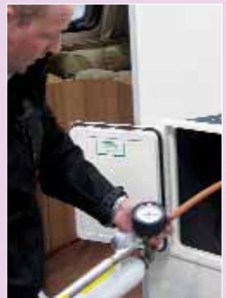
The gas supply system is checked for leaks using the standard air-pressure testing routine
