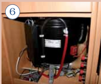
6. Trumatic combination heaters embrace space and water heating but they're bulky items
