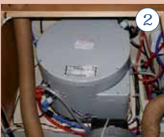
2. Water heaters often occupy a lot of space; this is the lower part of a wardrobe
