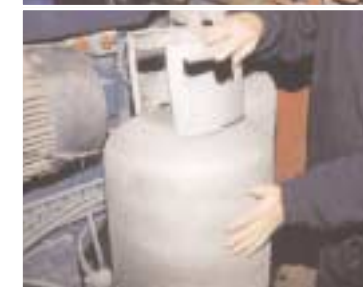
FROM THE TOP: A new base has been welded in place
